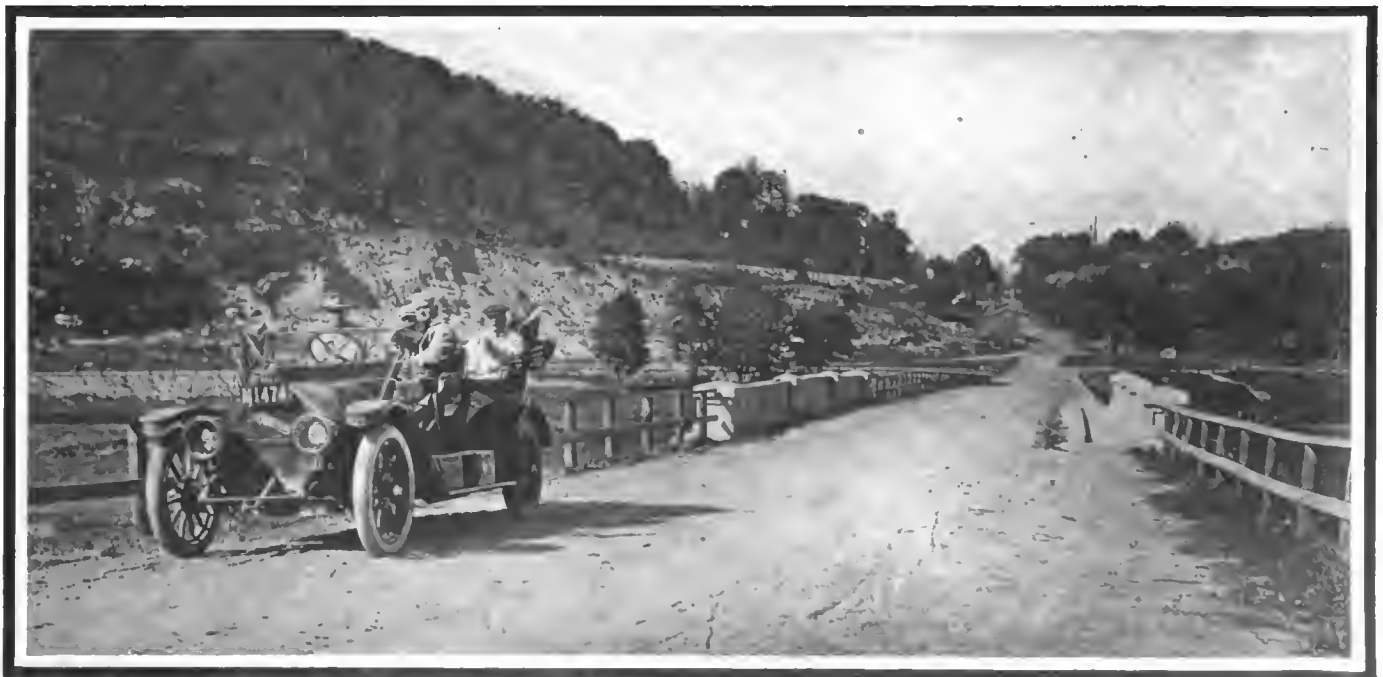
Fine example of New York highway crossing scientific culvert; note loose surface, which is practically dustless and easy on tires
